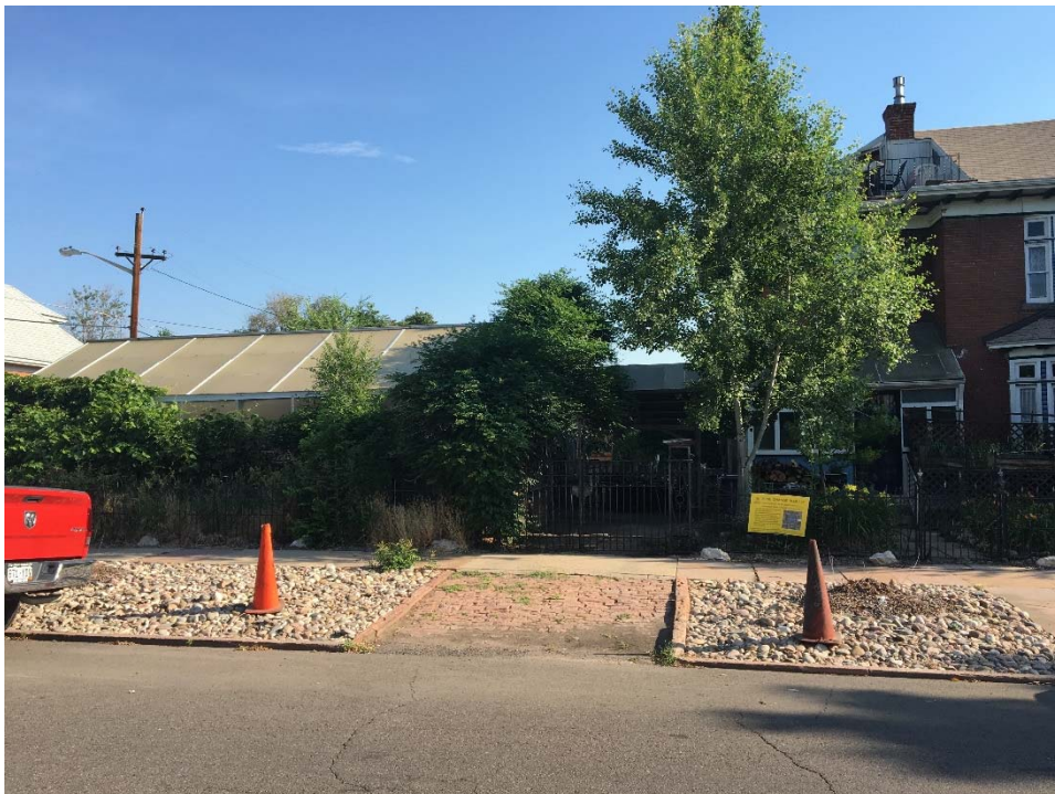
View of the subject site from 37 th Avenue, looking north. The carriage house/ former bake shop is located behind the greenhouse.
