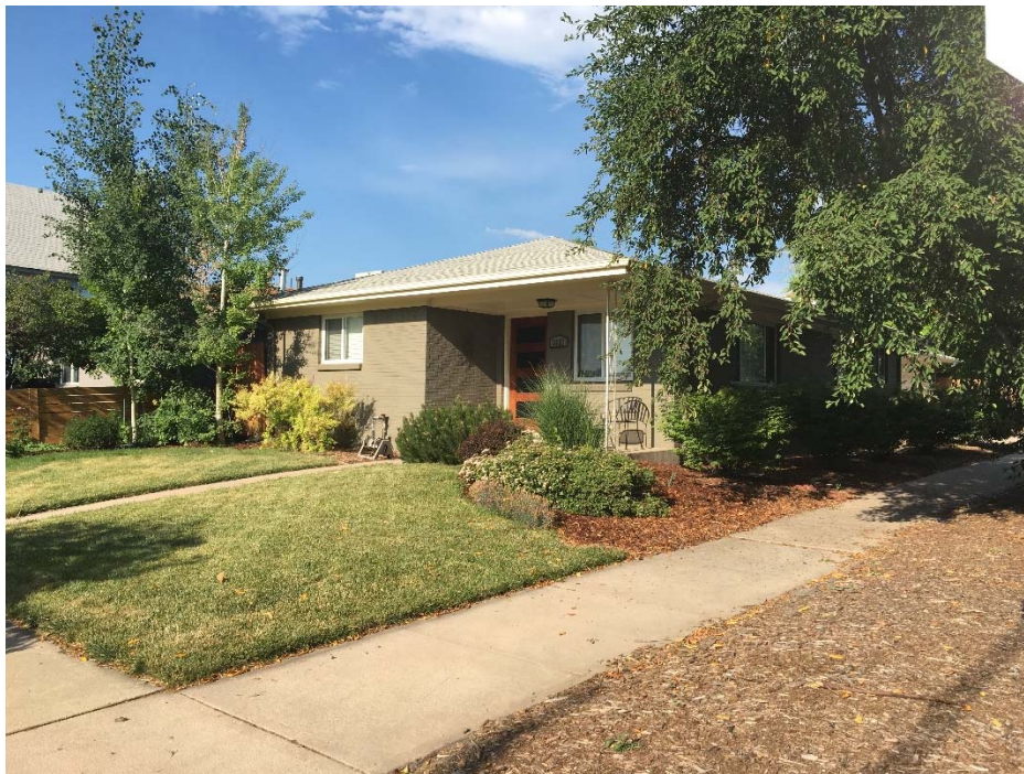
Single family home located south of the subject site, across 37 th Avenue and facing Shoshone Street.
