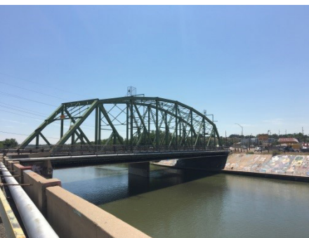
I-25/Ilex Truss Rehabilitation
