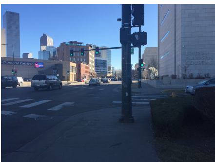
Colfax Curb Ramps, Denver, CO
