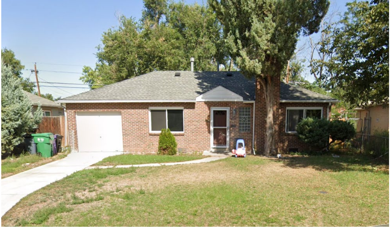
View of the property to the east, looking east.
