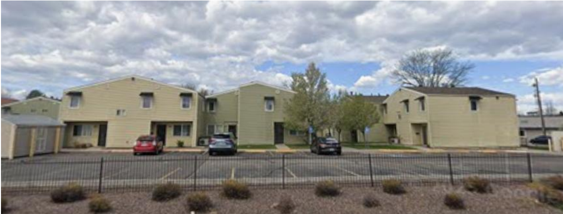
View of Multi-unit homes to the north of the subject site, looking west from South Monaco Street Parkway.
