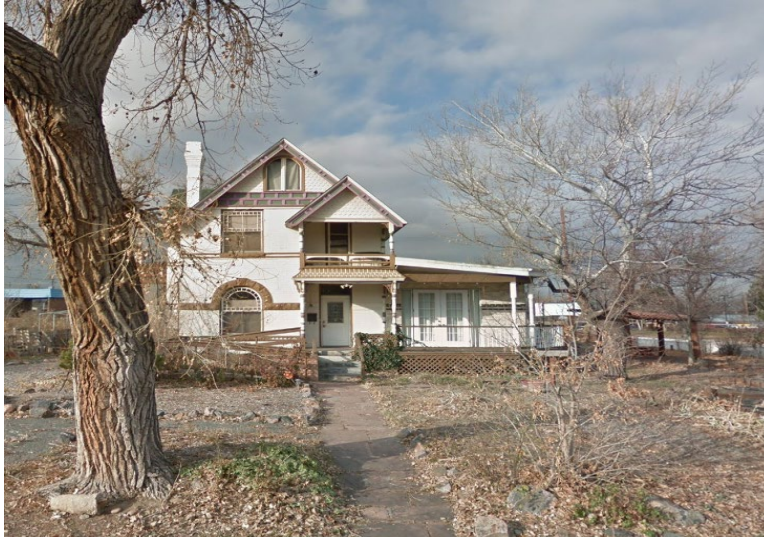
Subject site facing west from North Albion Street.
