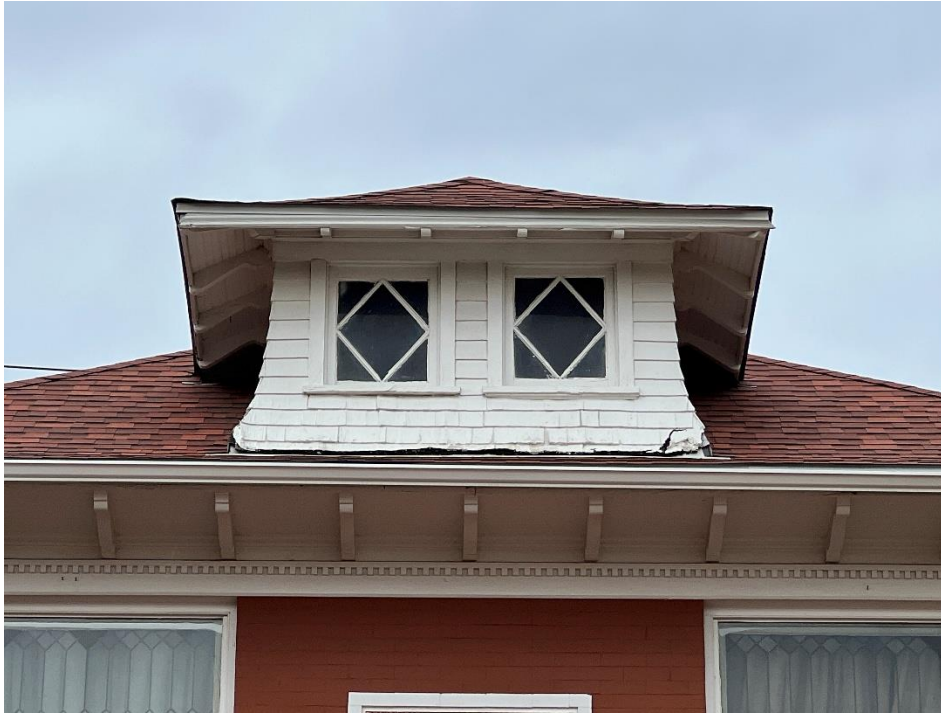
Photo 7. East elevation dentils and modillion details.
