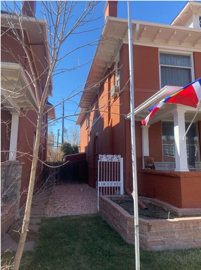
Photo 3. Southeast corner, South elevation.
