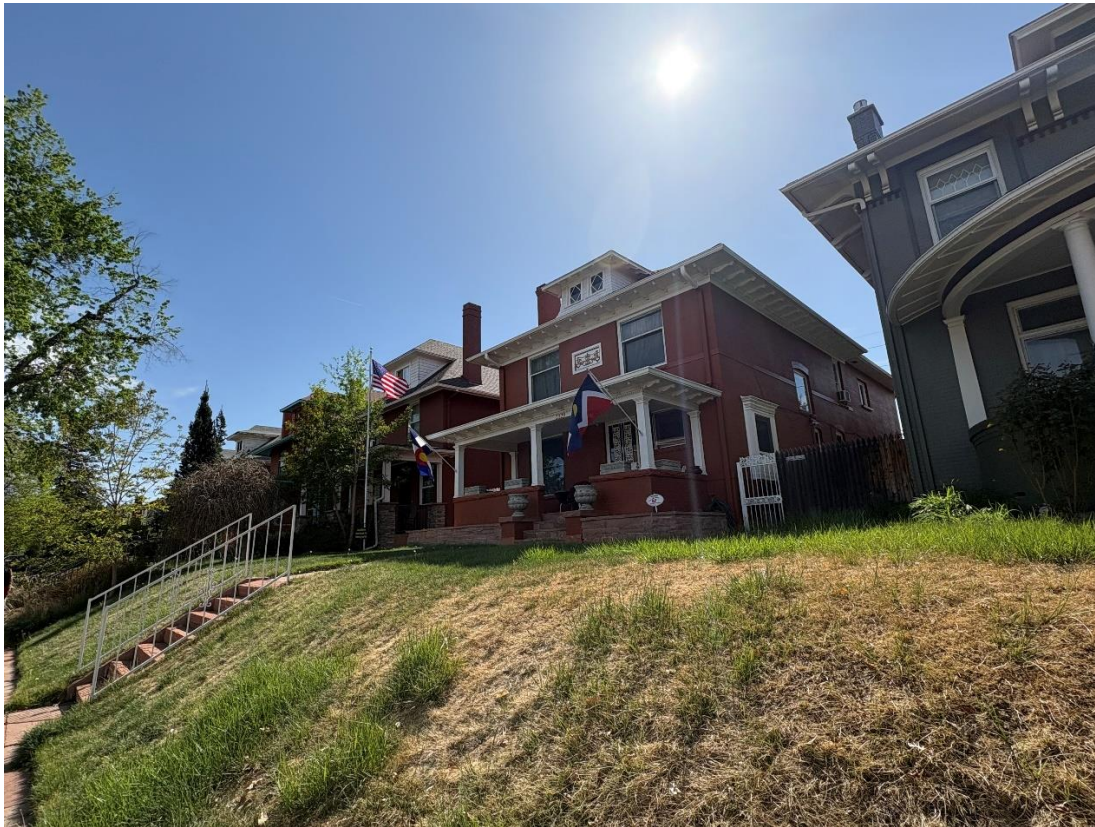
Photo 8. Overview showing east façade and adjacent residences.
