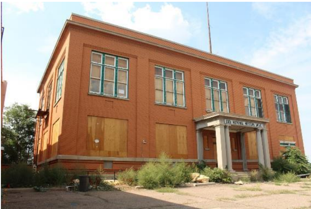
Figure 14. Former Armour Office Building, front (east) facade and side (south) elevation view facing northwest. 62
