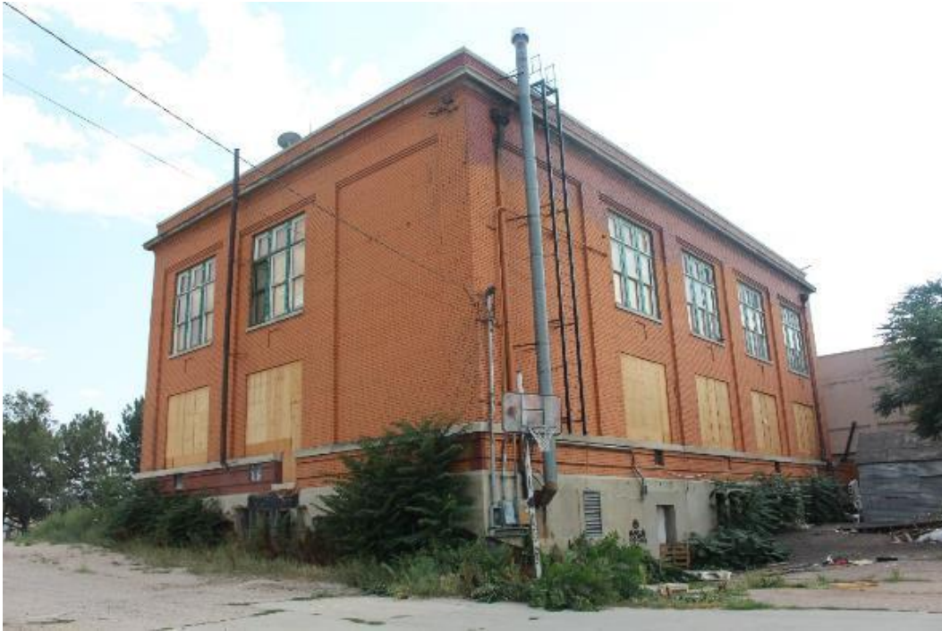
Figure 15. Former Armour Office Building, east and north elevations, view facing southwest. 63
