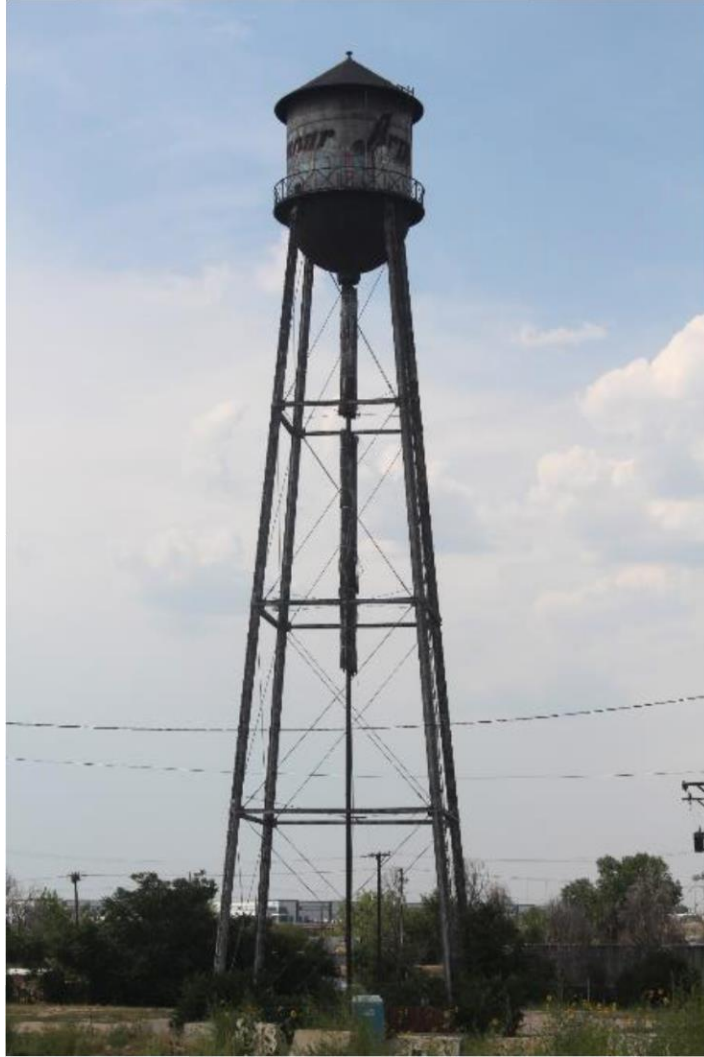
Figure 28. Armour Water Tower, view facing north. 73
