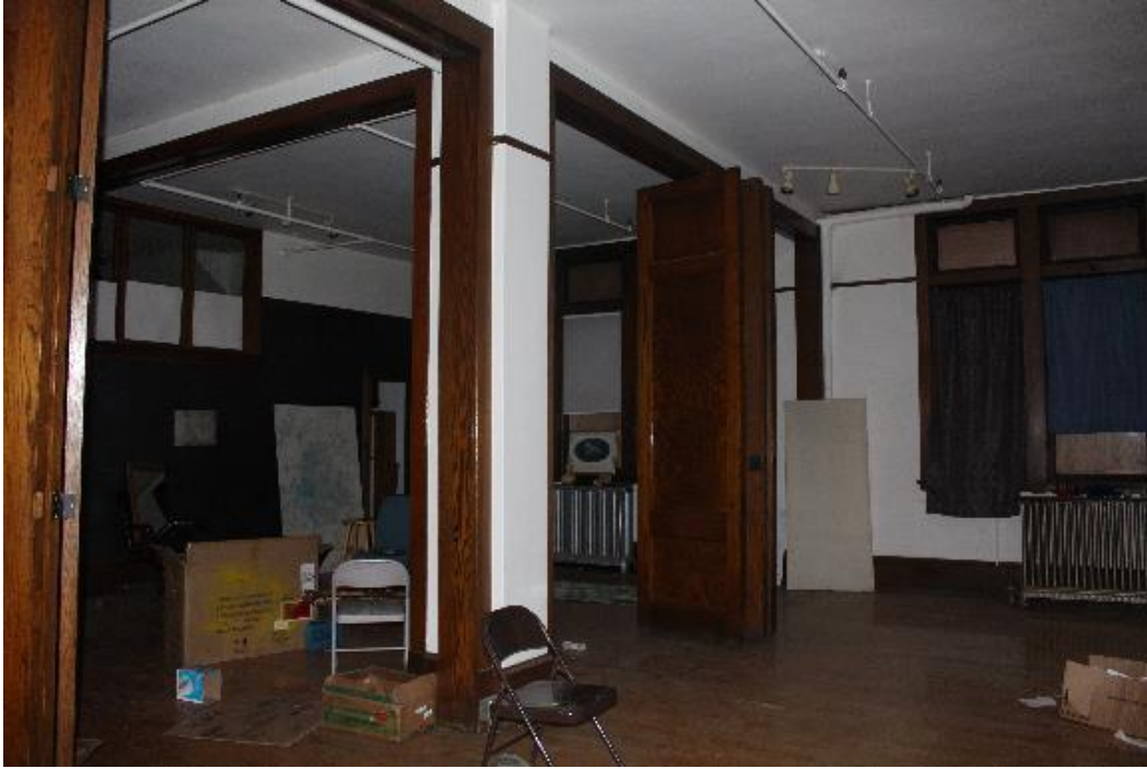
Figure 20. Interior view of full-height wood oak room dividers on the first floor. 67
