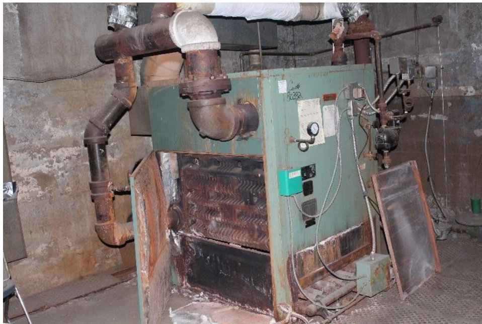
Figure 27. Original boiler in basement/cellar. 72
