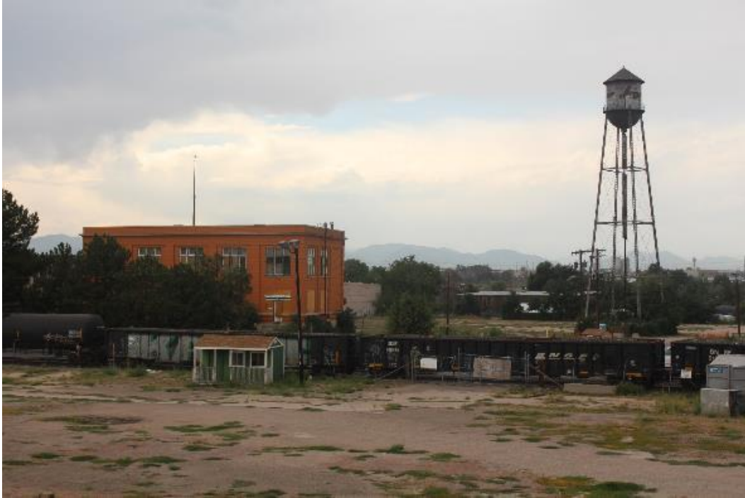
Figure 13. Overview of the Armour complex from the elevated walkway in the stockyards showing the former Armour Office Building and Water Tower. Note the noncontributing Ponderosa Pines that line the east boundary of the parcel and a train on the tracks currently operated by Denver Rock Island Railroad, which parallels National Western Drive. 61
