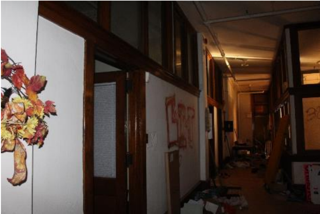
Figure 25. Original offices with wood doors and transoms on second floor. 70
