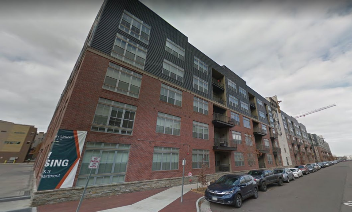
View of subject site from Huron Street, looking northwest.
