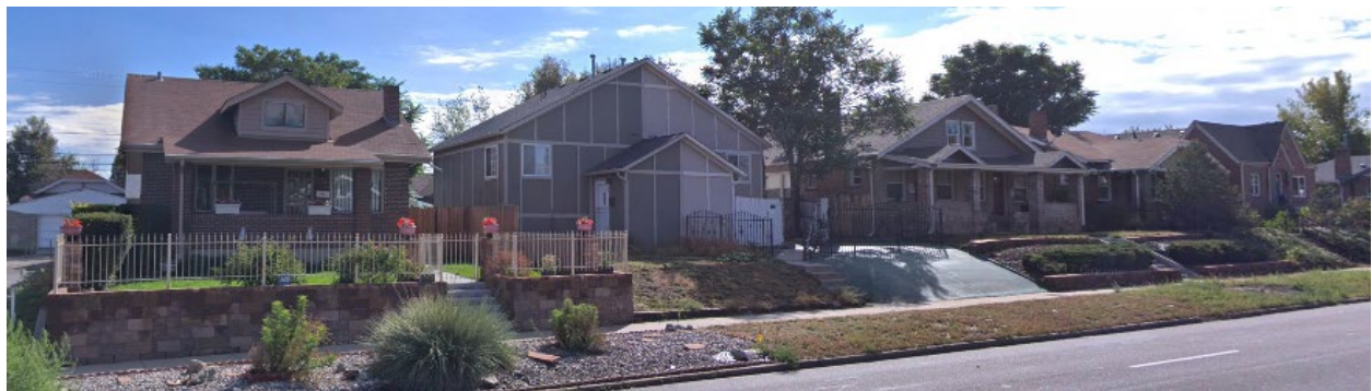
South - View of properties to the south, looking east from North York Street
