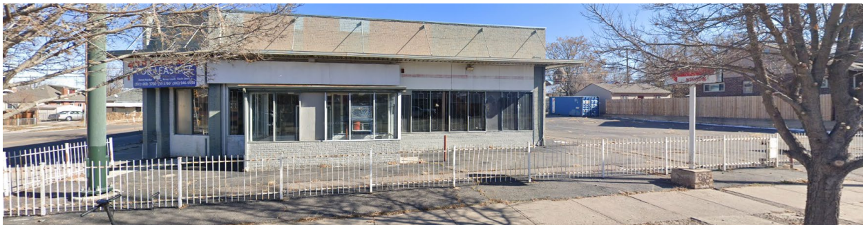
Subject Site - View of the subject property, looking east from North York Street
