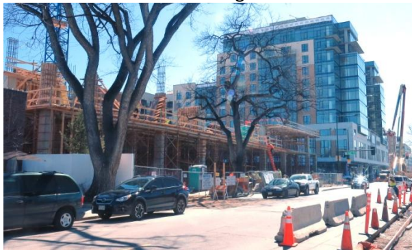
New 12-story construction on N Steele Street to the east and southeast of the subject site.
