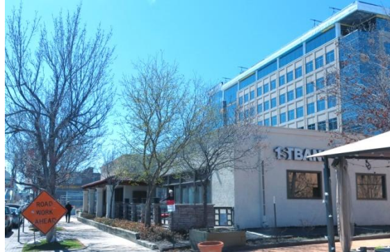
Subject site, looking south. 1-story bank in the foreground with new construction behind.
