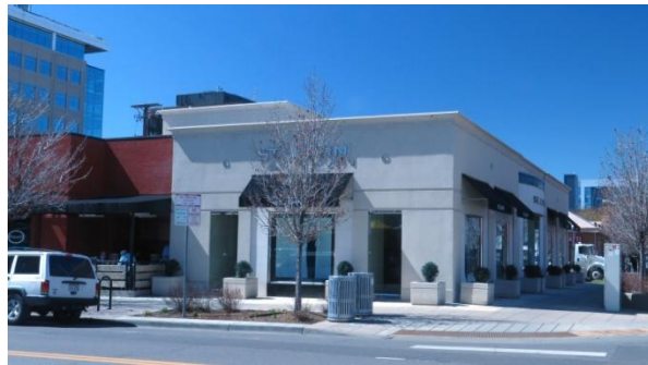
One-story commercial buildings on 2 nd Avenue to the north of the subject site.
