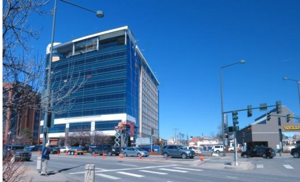
Subject site, looking north. 8-story, mixed-use new construction in the foreground.
