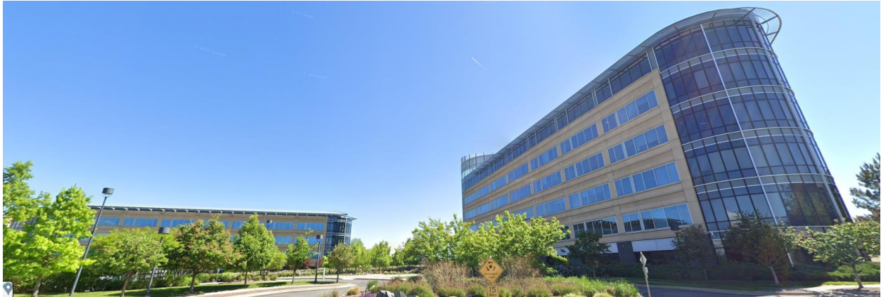
Google Image: View of the subject site looking northeast from S. Monaco Street.
