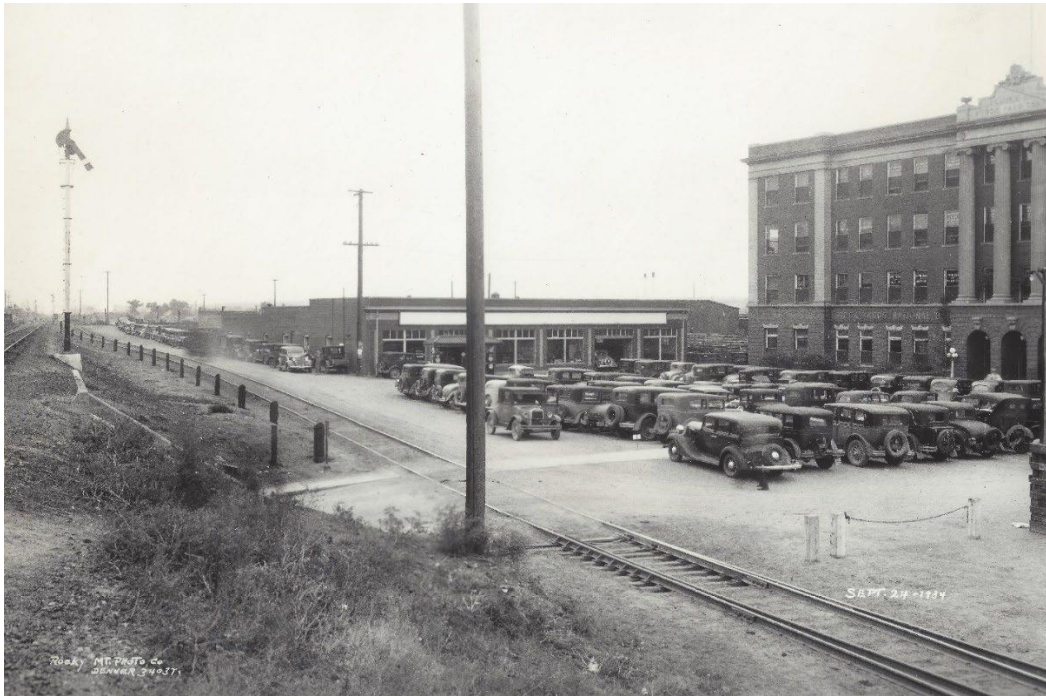
Figure 11. 1934 photo of Livestock Exchange and garage. The garage was constructed in 1917. The number of cars driven by those working in the Livestock Exchange compounded with freight trucks led to traffic congestion around the yards. Car owners dropped their keys with attendants in the garage with instructions to fix or maintain their cars while they were conducting business in the yards. 44
