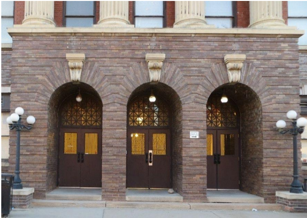
Figure 1. Front (southeast) entrances of the 1916 structure with large arched transom. 5
