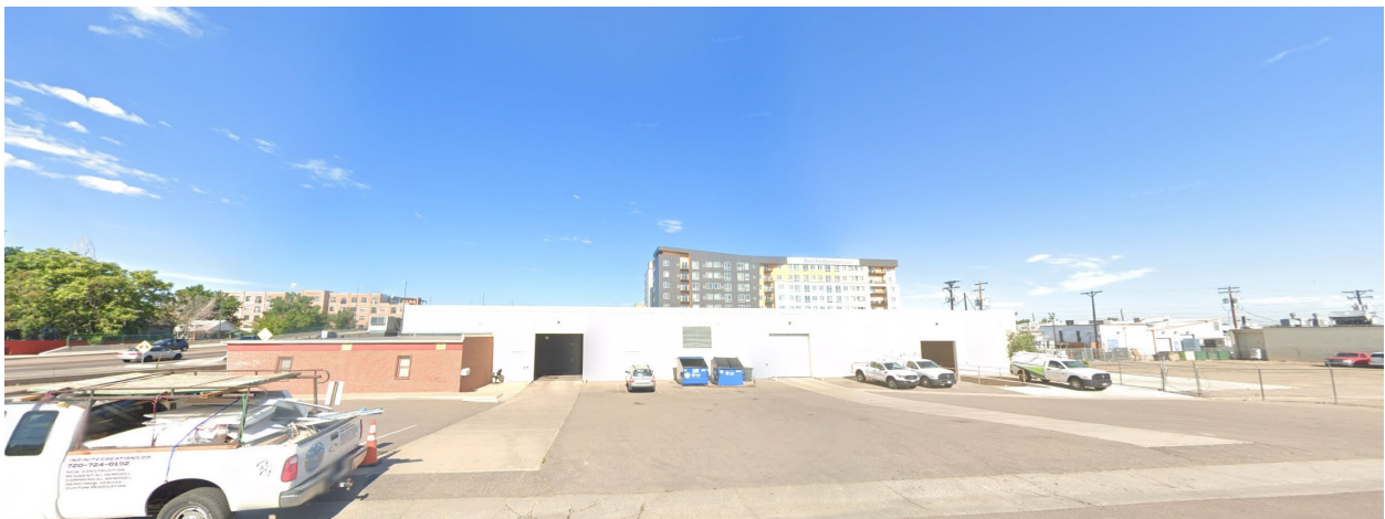
West – from South Bannock Street, looking west
