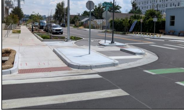
Safer Intersections - Bulb-out
