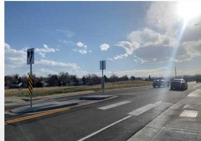
Maxwell Elementary Pedestrian Improvements
