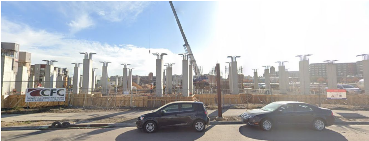
Site – from Denargo Street (Source: Google Maps)
