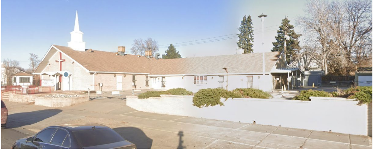
View facing east on Colorado Boulevard south of 26 th Avenue
