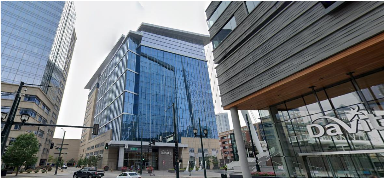
The property to the west across 16 th Street, facing west.
