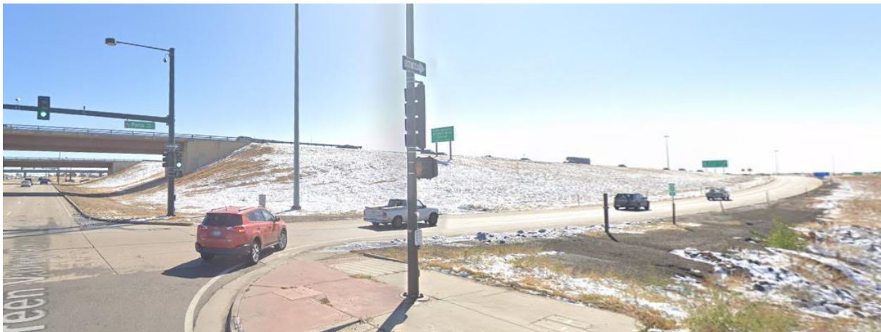
View directly east of the site of Pena Blvd, looking south from Green Valley Ranch Blvd.
