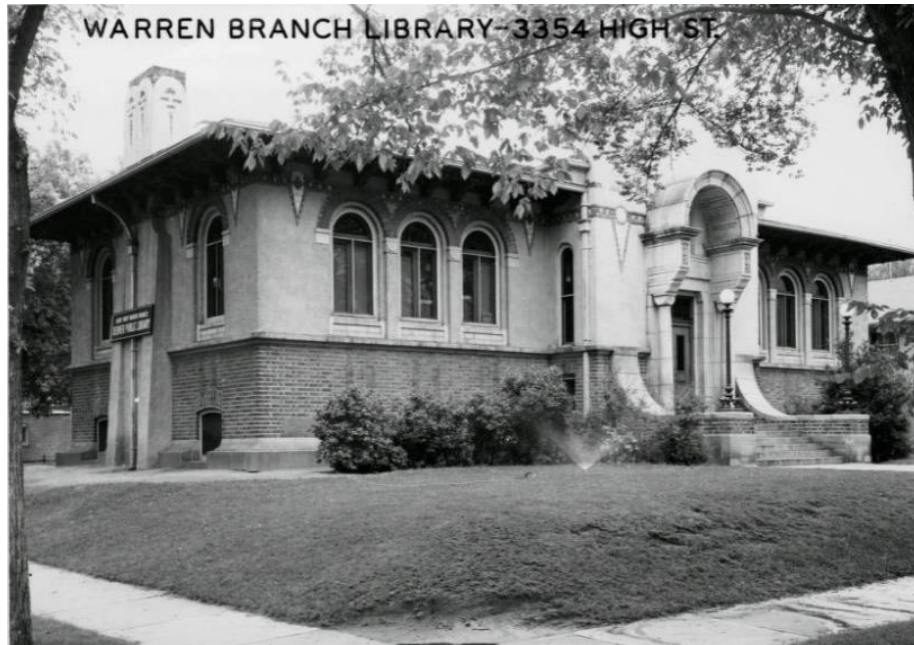
Figure 12 - The Warren Branch Library at 3354 High Street. Denver Public Library Digital Collections.
