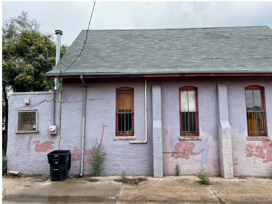
East Facade of 1618 E. 38 th Ave.
