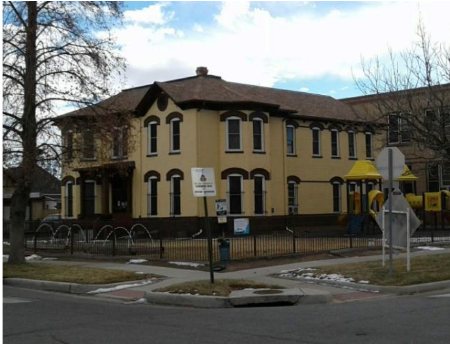
Figure 2 - The Amos and Sarah Bissell house, located at E. 36th Avenue and Lafayette Street, is now the office for the Annunciation Catholic Parish. The house was constructed around 1885. Discover Denver photo.
