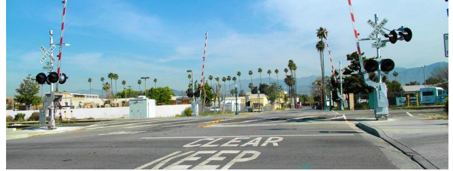
Quad-gate installation
