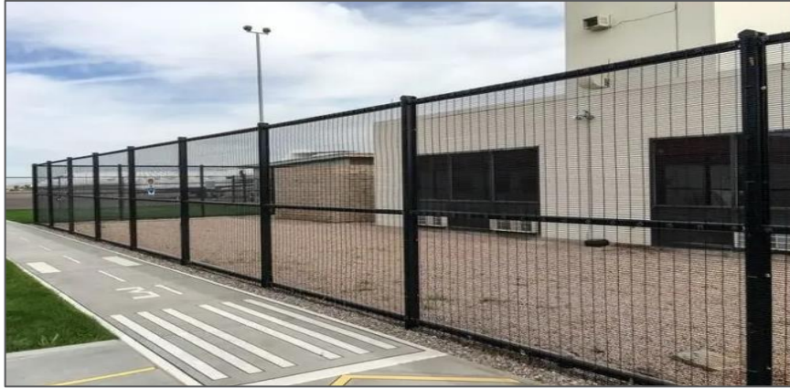
Anti-climb fencing to prevent trespassing
