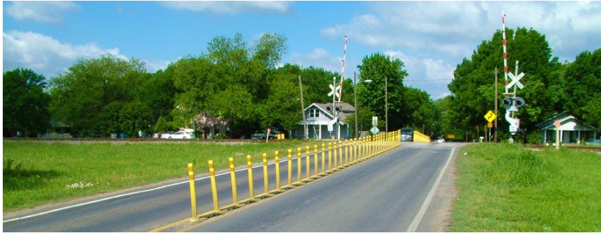
Two-gate with roadway channelization
