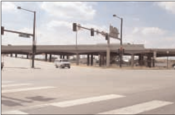
Construction is nearing completion on the I-70/Brighton intersection, an "event" that is likely to stimulate development
