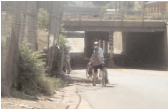
Safe and convenient bike access, such as fixing this missing bicycle link along 38th Street, is recommended by the Plan
