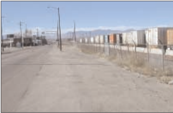
40th Avenue and drainage needs have been studied recently
