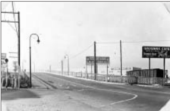
Broadway viaduct, circa 1930
