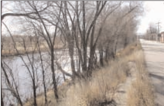
Part of the 50-foot Ringsby Court right-of-way is taken up by the bank of the river making it difficult to provide sidewalks and other amenities
