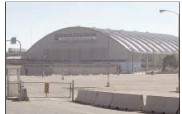
The Denver Coliseum is in the Events District
