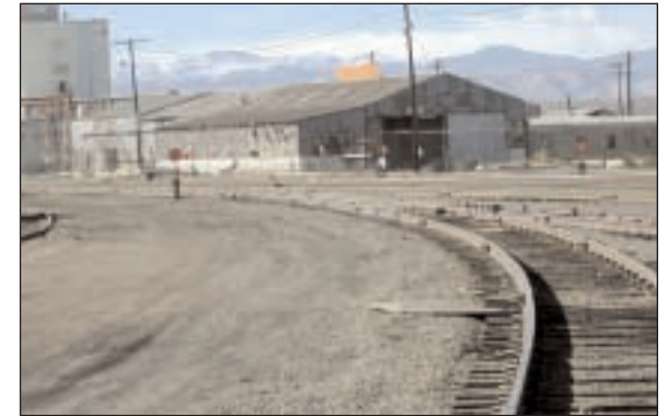
The vicinity of 40th Street and 40th Avenue, is a potential rapid transit station location
