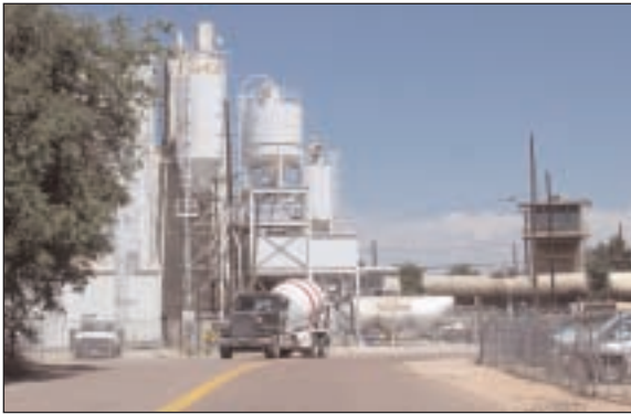
This concrete plant is an allowed use under the existing industrial zoning
