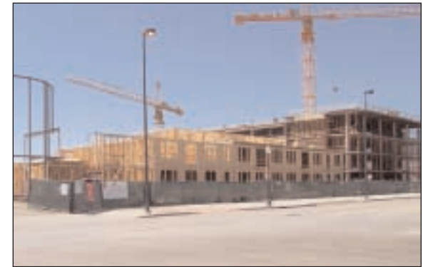
JPI is constructing 241 apartment units along Brighton Boulevard
