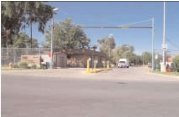
RTD facility on Ringsby Court
