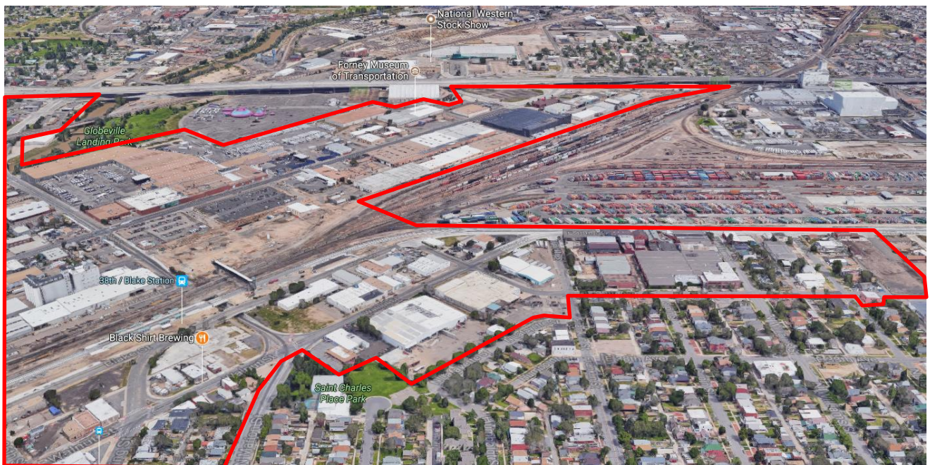
This image shows the northern half of the study area looking north with Franklin Street located north-south at center-right.
