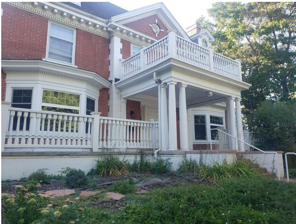
1741 Gaylord Street, front façade
