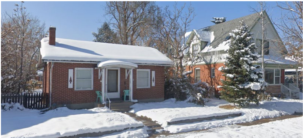
South - View of the properties to the south.
