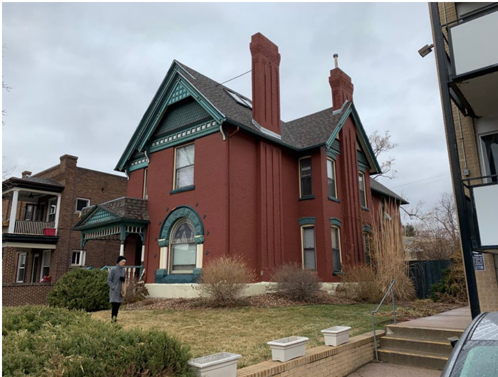
Photo of west and south facades of 1272 Columbine Street (Scott Crotzer, 2020)
