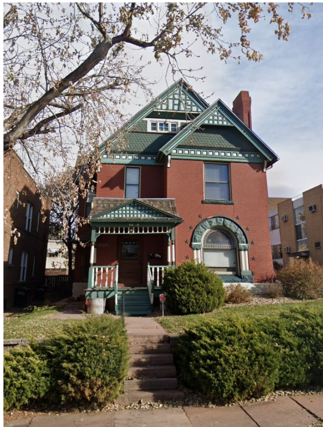
Photo of west facade of 1272 Columbine Street
