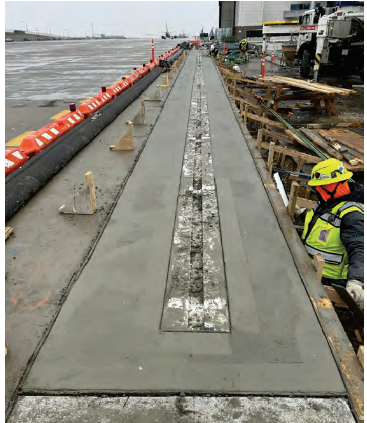
Figure 12. GARDI A-SE Self-Performed Trench Drain
