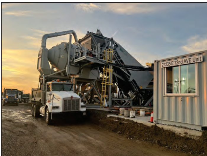
Figure 5. MW Central Mix Batch Plant - DEN
