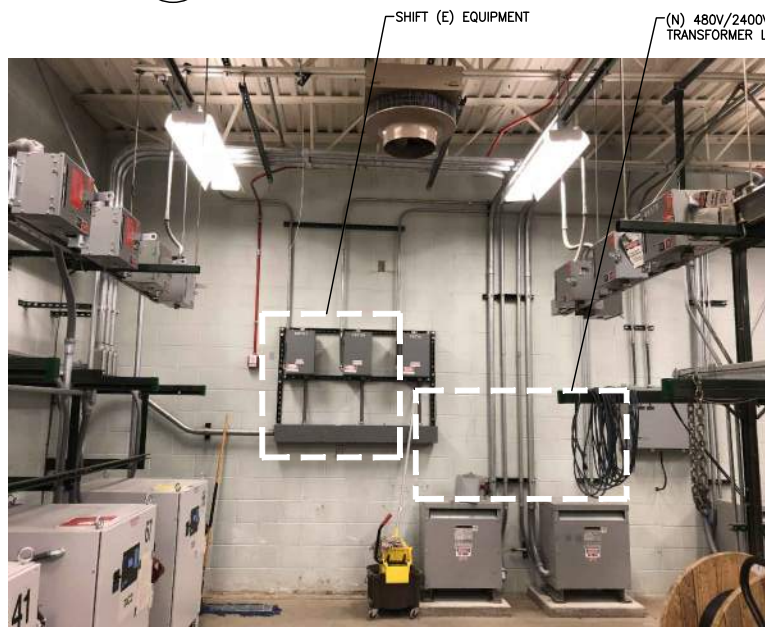
1 ELEVATION VIEW OF 35LCP1 & 35LCP2 TRANSFORMERS & CUTOUTS NOT TO SCALE
