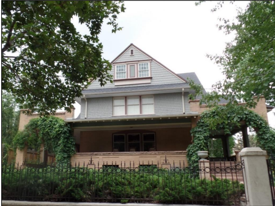
670 Marion Street, front façade
