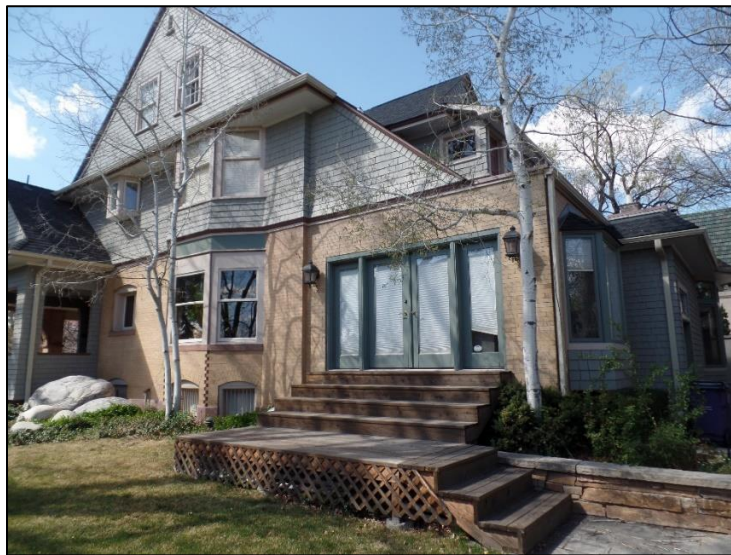
670 Marion Street, side and rear elevations
