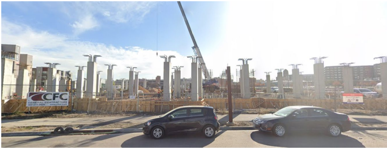
Site – from Denargo Street (Source: Google Maps)
