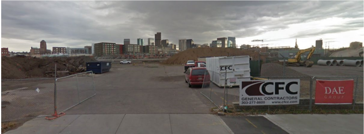
Site - from Wewatta Way (Source: Google Maps)
