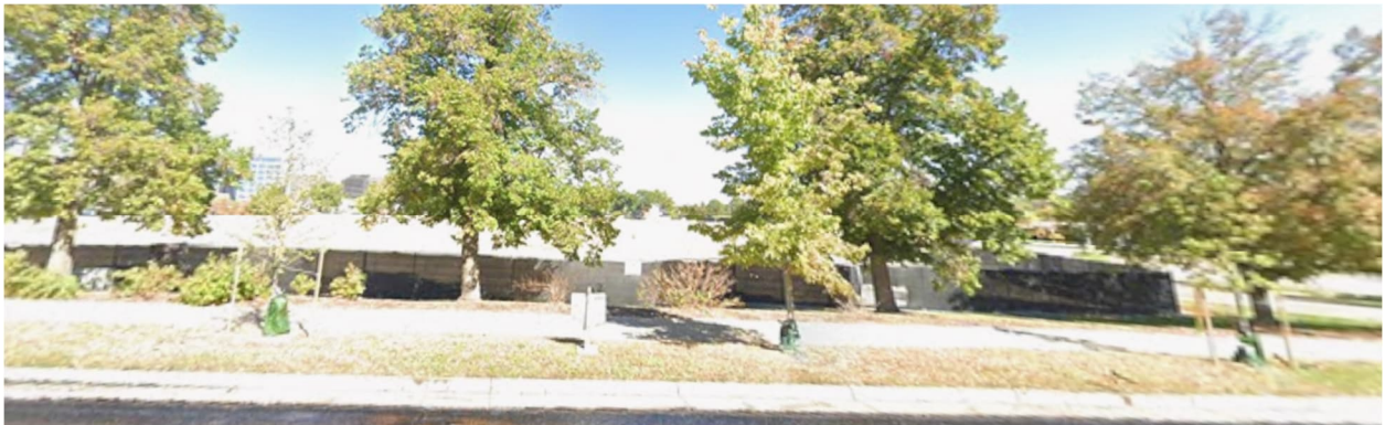
View of the under-construction property to the west from East Belleview Avenue looking north
