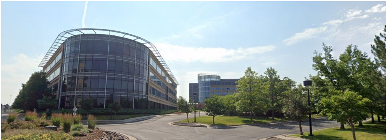
Google Image: View of the subject site looking southeast from S. Monaco Street.
