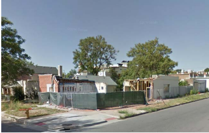
Site – at 37 th Ave. and Mariposa St.
