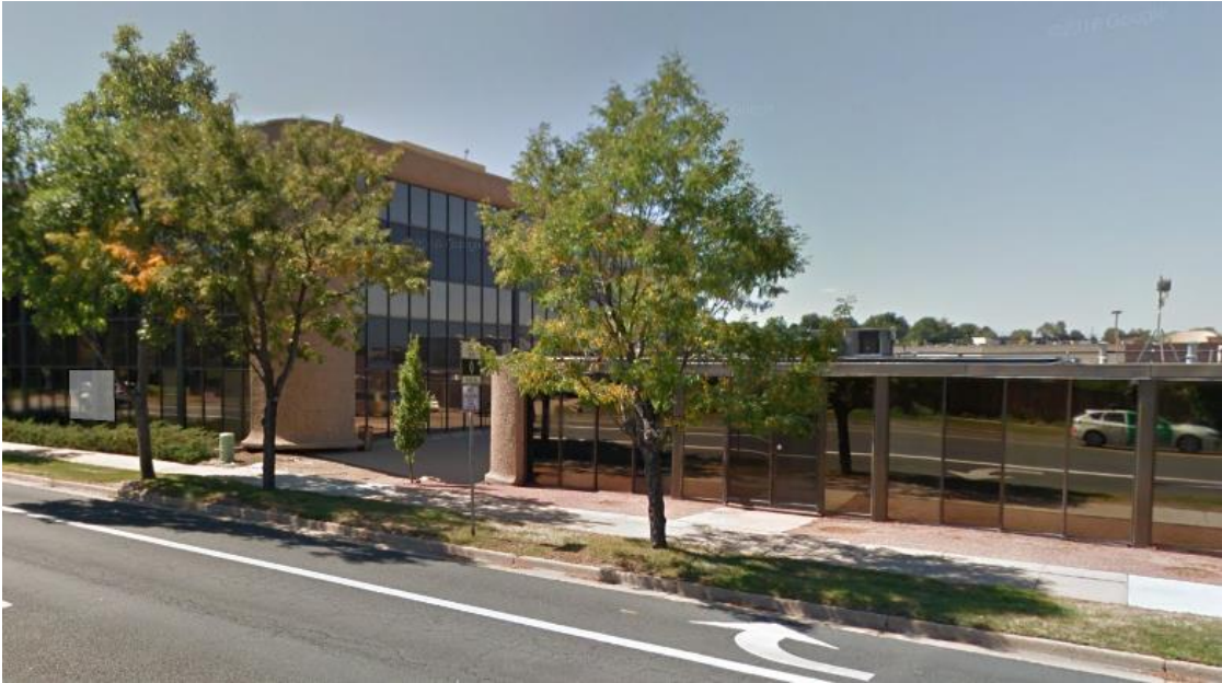
Subject Site, looking west
