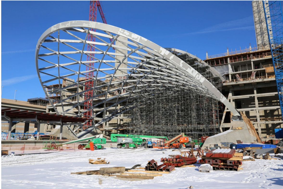
Placement of Train Canopy Steel
