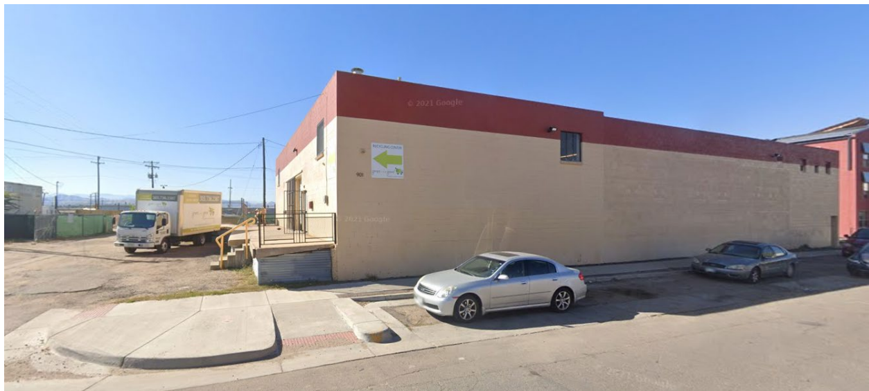
Site: Looking west from Navajo Street (Source: Google Maps)
