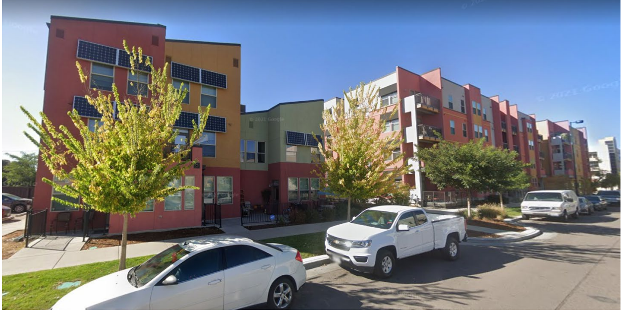
North of site: Looking west from Navajo Street (Source: Google Maps)
