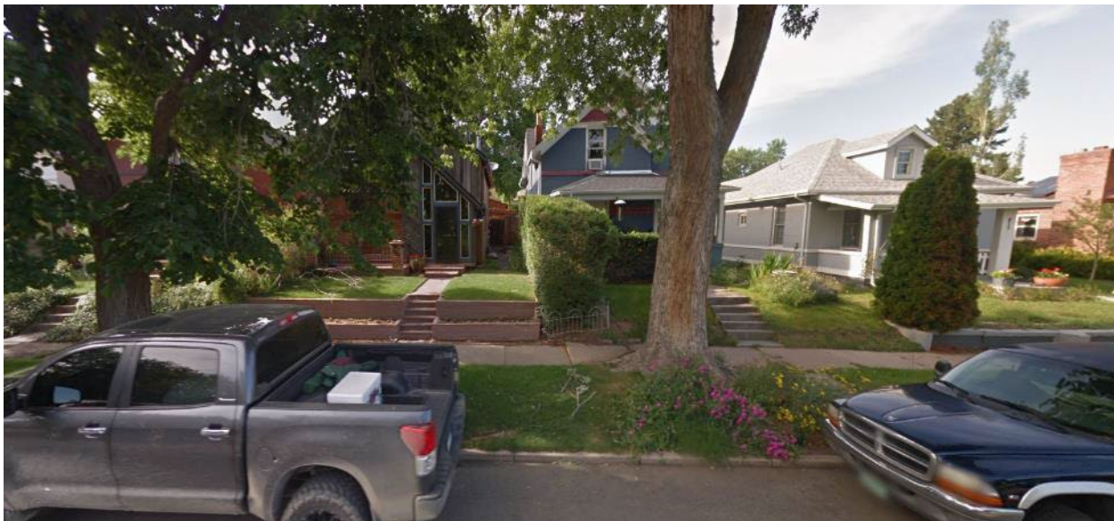
View of the subject property looking north.
