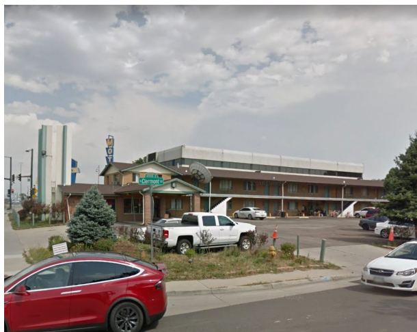
Site – from Clermont St. & Evans Ave.
