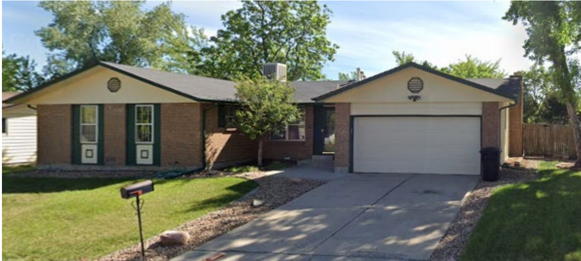
View of the property to the north looking east.
