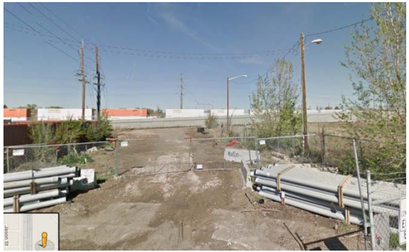
West – BNSF Rail right-of-way corridor.
