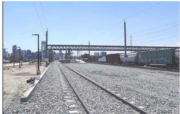
Recently constructed pedestrian bridge at the 41 st and Fox Station platform construction site (Source: RTD)
