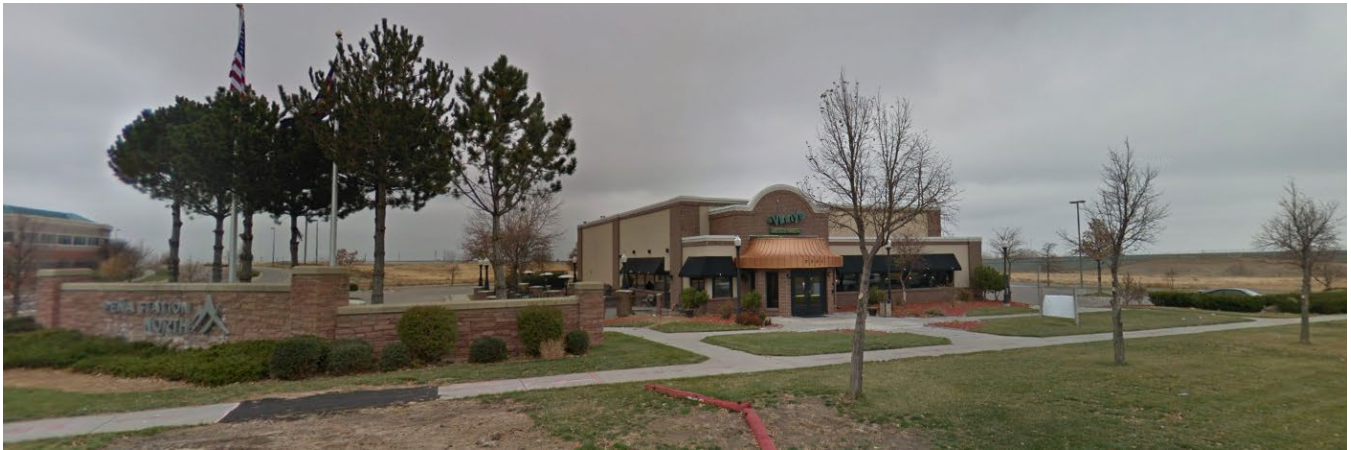
View of the subject property on Tower Road, looking west. (Source: Google Maps)
