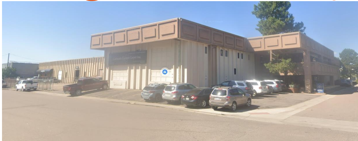
Subject property looking southwest
