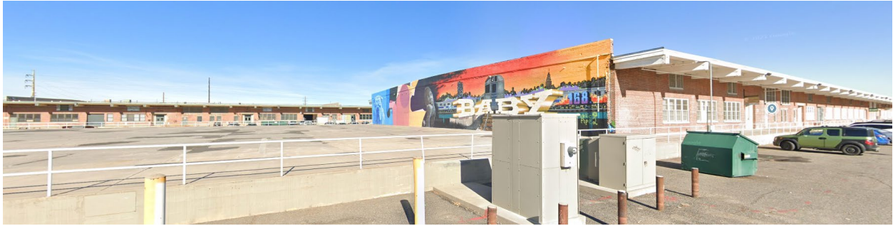
South - View of the York Street Yards properties from the south, looking northeast.
