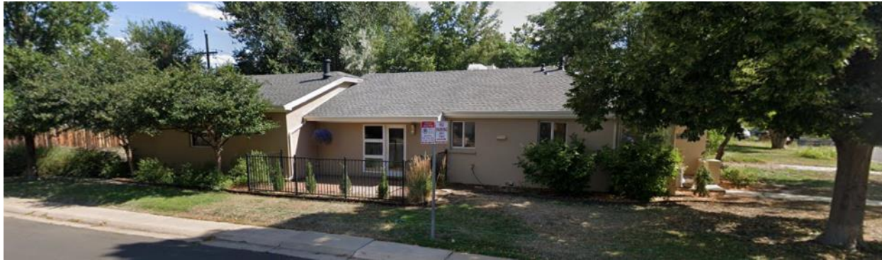
Single unit home to the south
