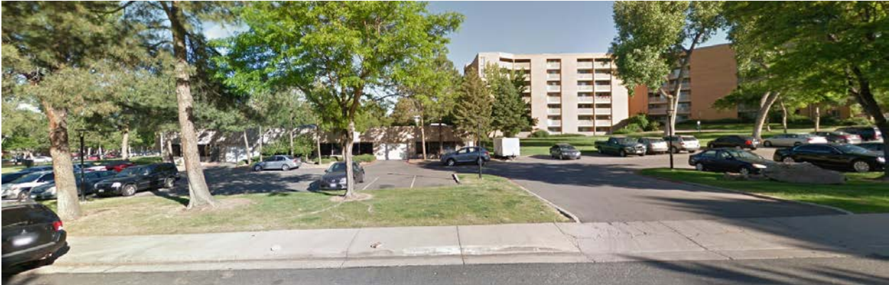
Woodstream Village Looking West
