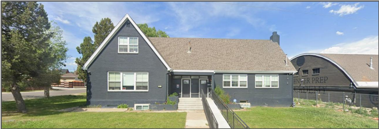
View of the subject property looking west from South Zuni Street.
