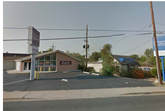
Commercial/retail and office located on southwest corner of Exposition and Leetsdale.
