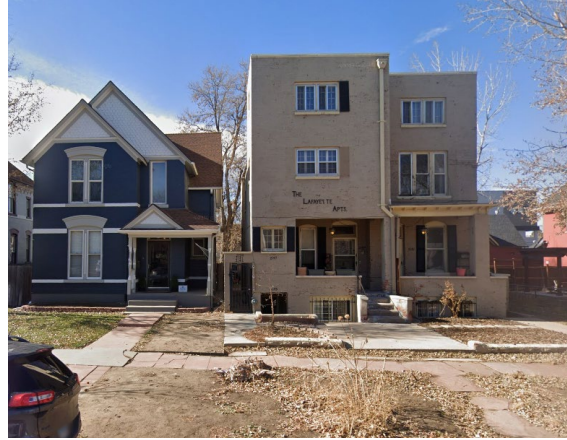
South – from Lafayette St.
