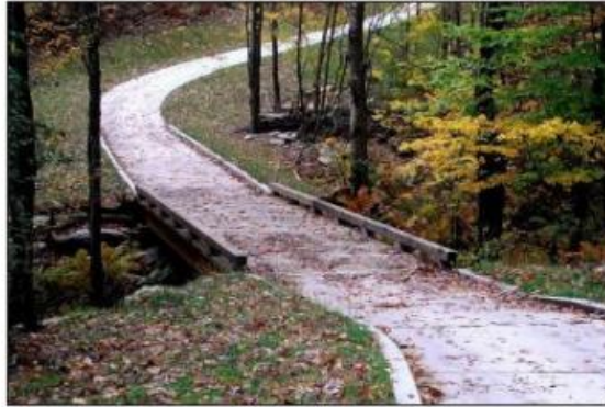
Cart Path Bridge (City Park hole's: 6, 7)
