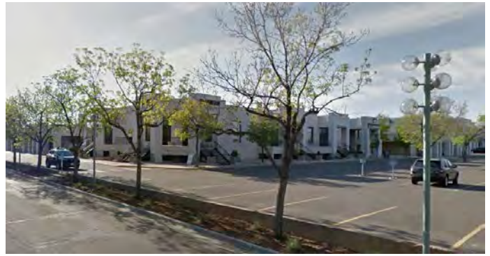
One story retail/office structure to the east of the site
