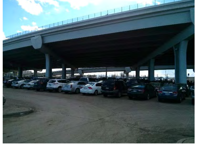
Subject site looking south
