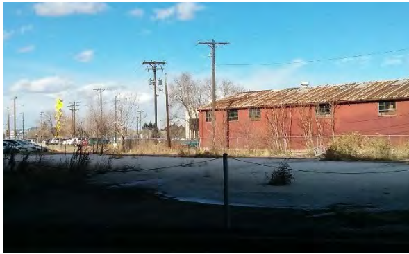
One-story warehouse to the east of the site
