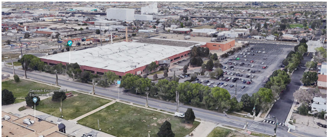
Subject property, looking northwest
